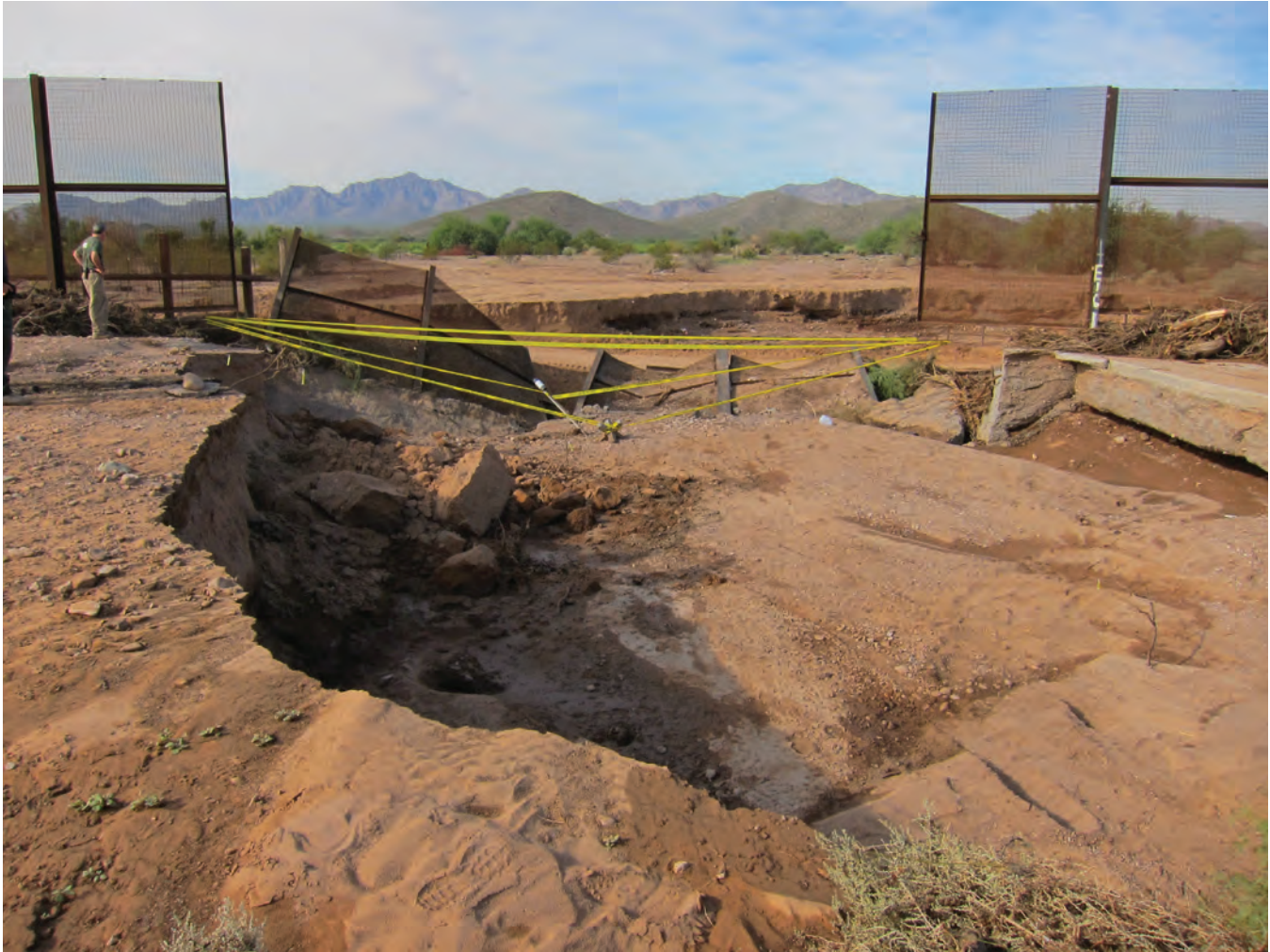
Organ Pipe Cactus National Monument shows the erosion caused by torrents of water redirected when heavy rains trap debris against a border wall.
